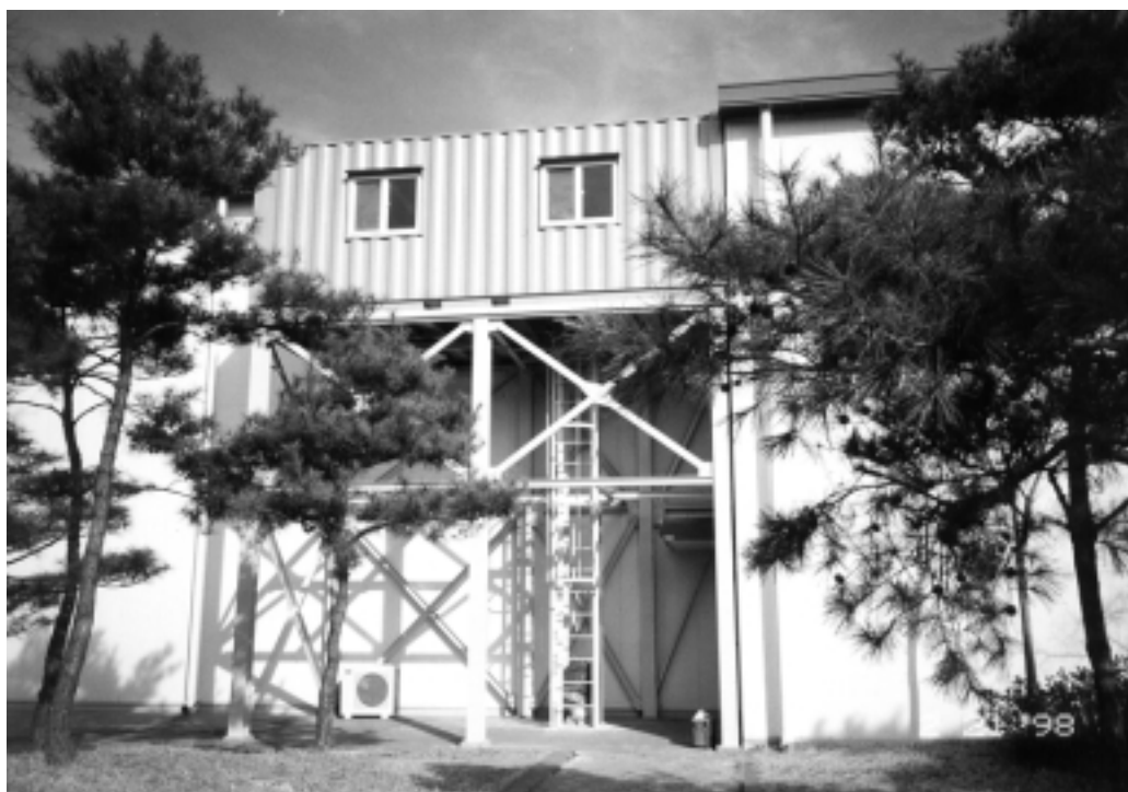
Fig. 4. Picture of constructed TOF facility
